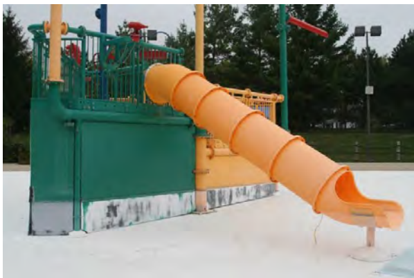
Faded paint on feature
