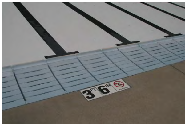
Existing rim flow coping
