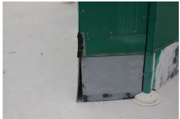
Tape holding feature corner/gap
