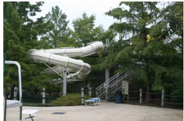
Existing slide tower access
