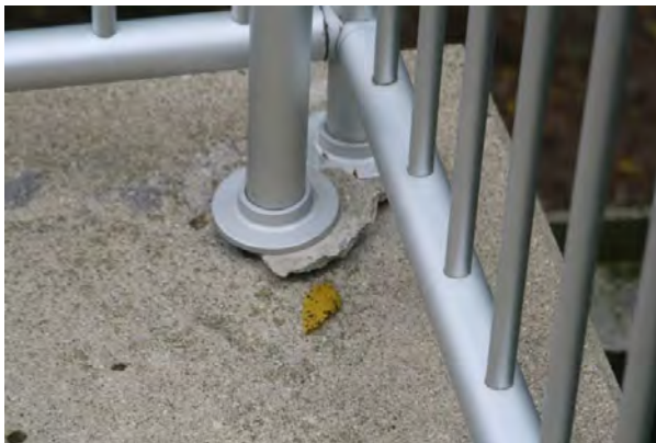
Concrete spalling
