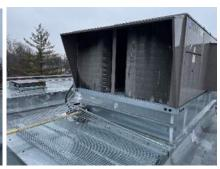
Existing YORK units on north end of building. Condenser guard to be installed on east unit.
