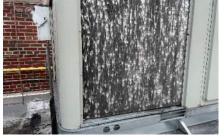
Severe hail damage on TRANE Unit 2.
